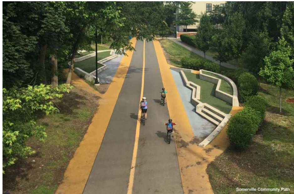
Figure 15: Example from Mass.gov of a Shared Use Path with Separate Bicycle and Pedestrian Lanes
