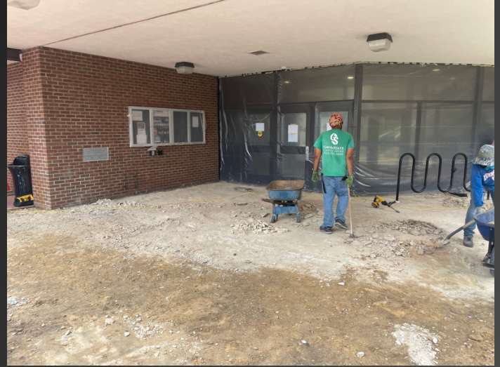
University Brick Paver replacement.
