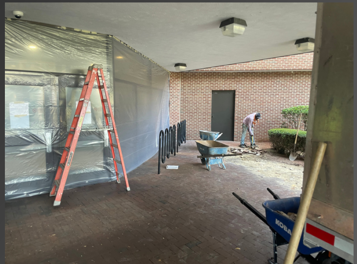
University Brick Paver replacement.
