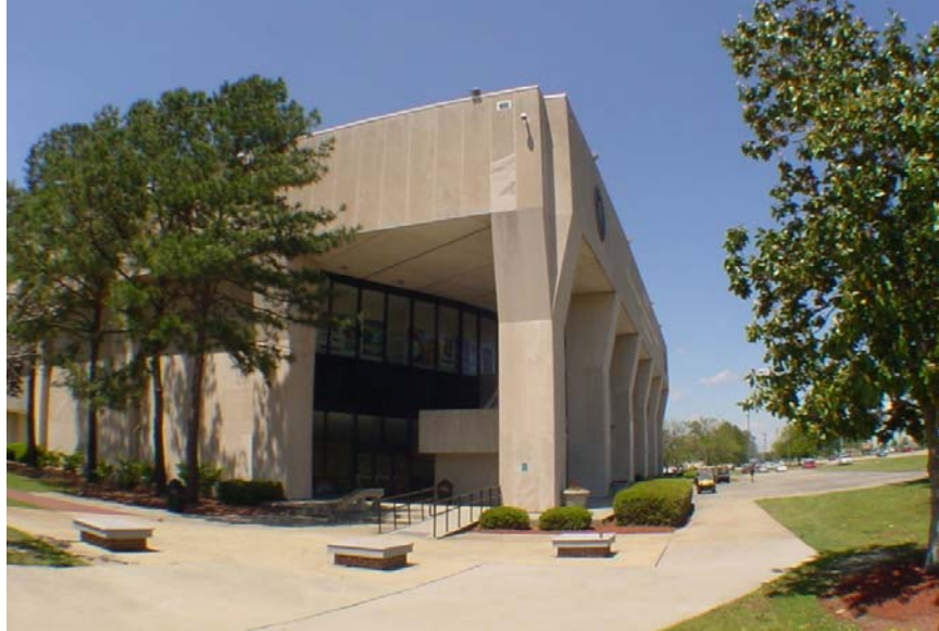
Southeast corner, with undersized lobby
