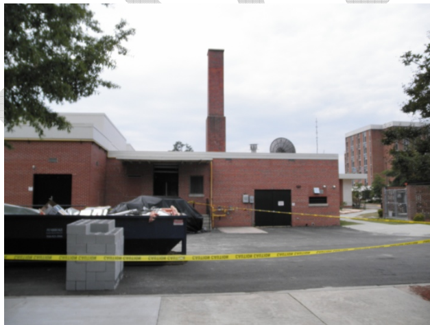
North Elevation of Lowry Building needs screening from Information Commons Building
