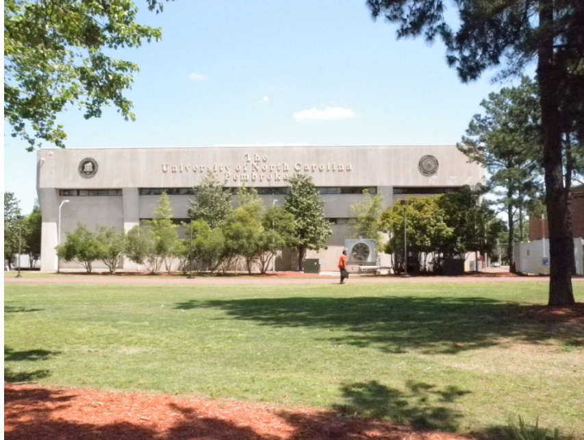
West façade has poor relationship to campus green space.
